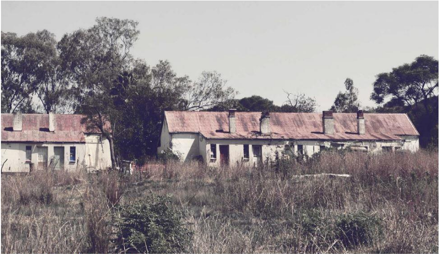
Illustration 1: Housing complex at Fort West in Pretoria West (Author, 2012).
